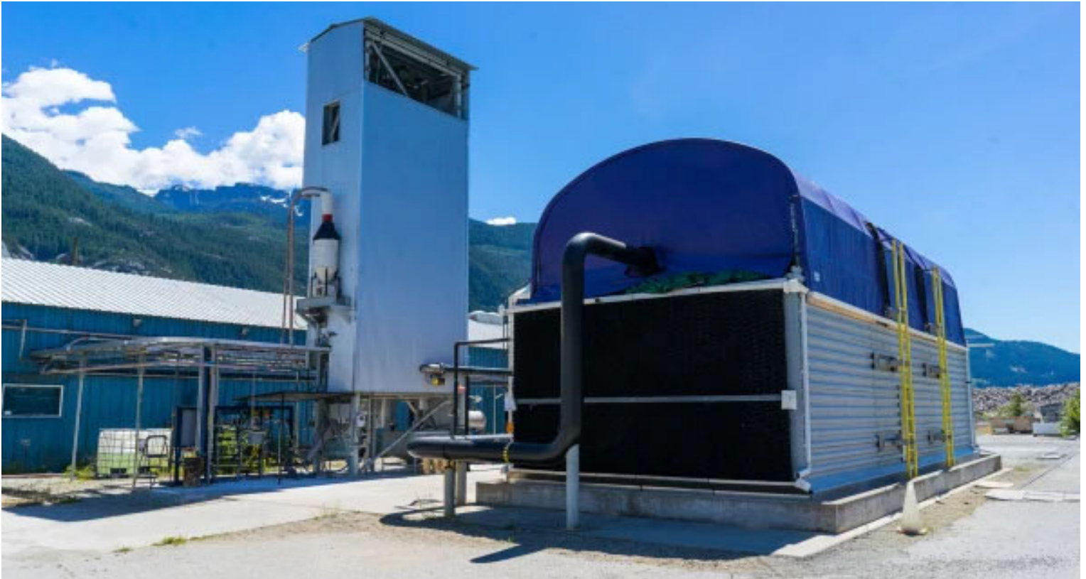
Climate Engineering’s direct air capture pilot plant in Squamish, B.C. [Photo: Carbon Engineering]
